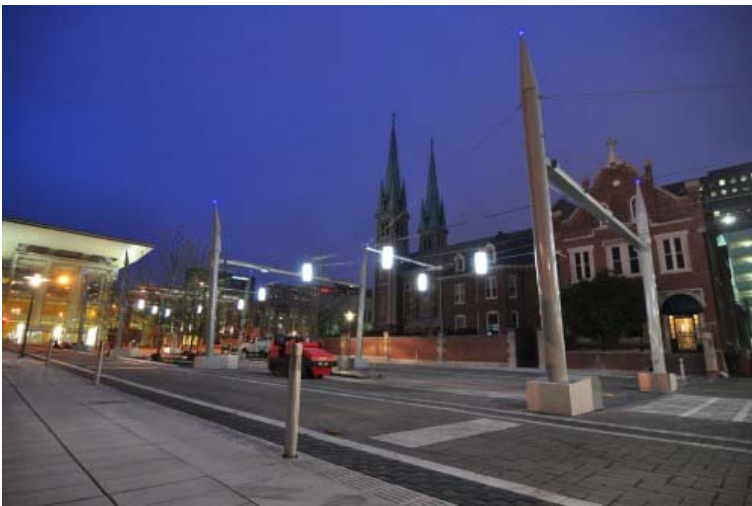
Georgia Street during construction (image credit: Curt Ailes)
