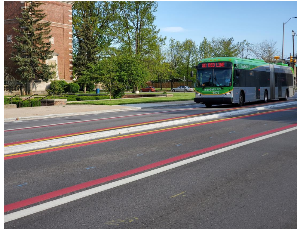
Center-Running Dedicated, Bus Only Lane
