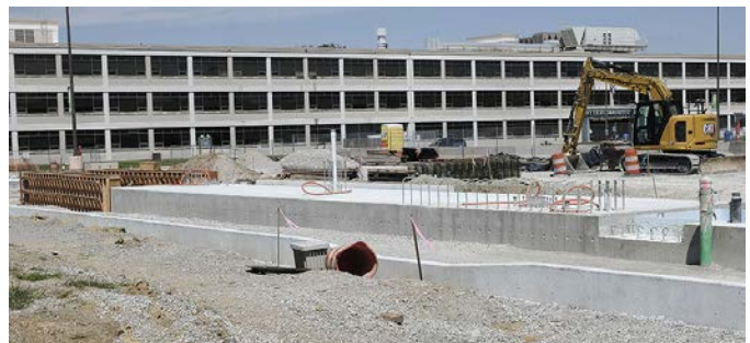
Above: Purple Line construction
