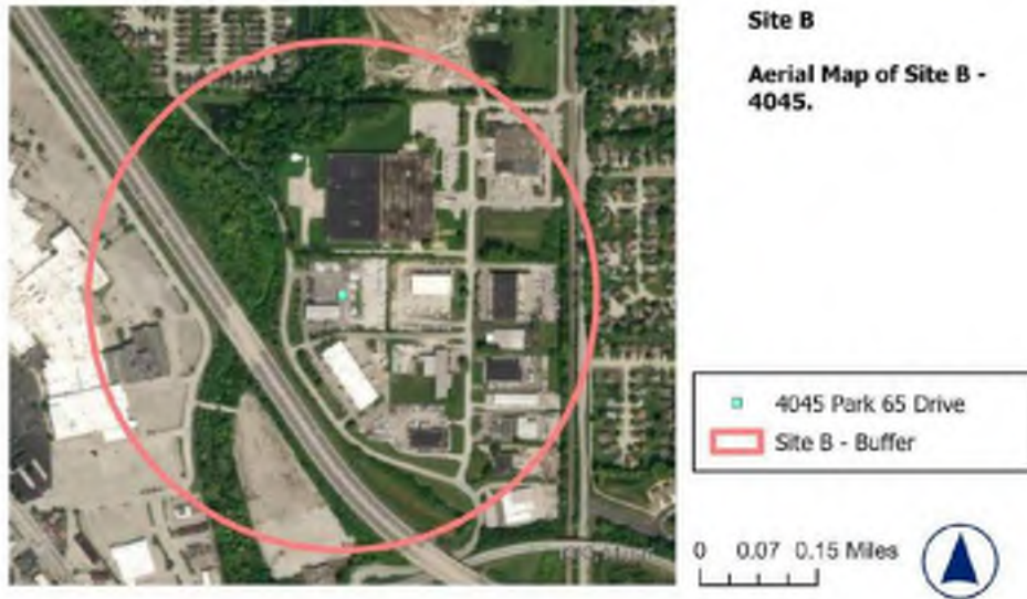
Figure II-2. Aerial Photograph of Site B
